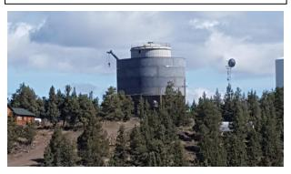
painting the tank at ground level. This part of the project will take about 12 days. During the painting process the crews hours may very depending on the weather and the winds. In order to apply the paint and coating correctly the wind, temperature and humidity have to be just right to ensure the paint bonds properly.
