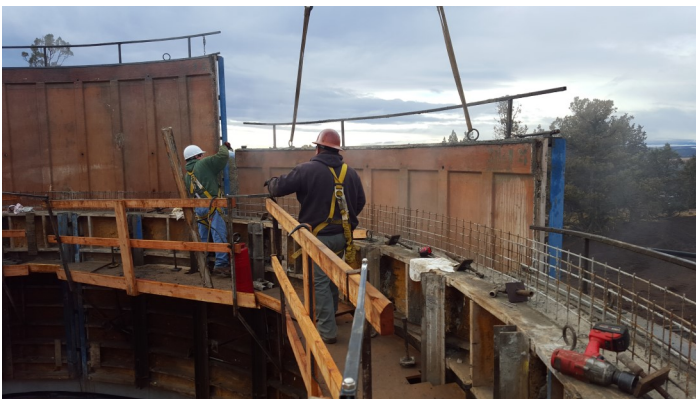
Landmark crew working to set the forms for the third lift. There is a total of 10 lifts to complete the pedestal.
