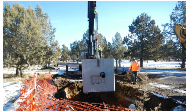
JRS crew placing the PRV Vault on the corner of Meadow and Peninsula.
