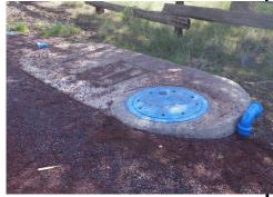
3 feet by 5 feet. This makes accessing and maintaining the equipment safer and easier. It also allows for an easy form of exit in the event of an emergency. These lids are also lockable and can only be accessed if you have a special tool.
